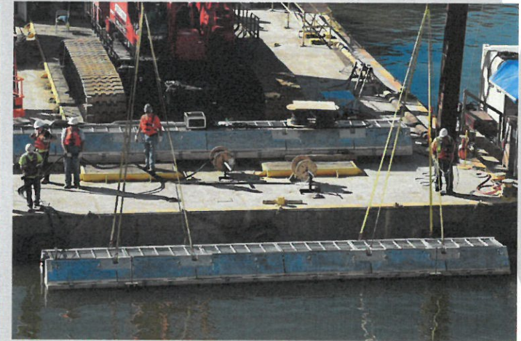
Above – Bioacoustic barrier installation at Barkley L/D, KY
